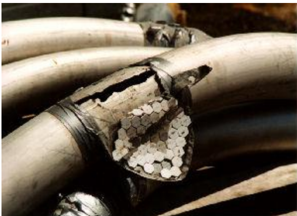
A common sight at RheTech before the HammerTek Smart Elbows were installed was an attempt at patching with ceramic tiles and duct tape.
